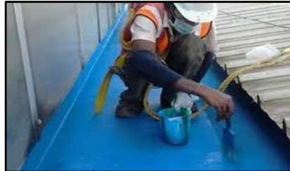
FRP Surface Treatment & Lining Service
